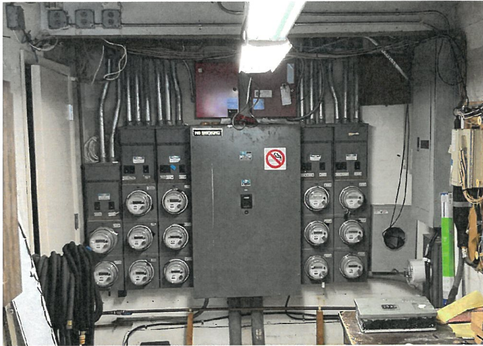
Electrical Systems Installed
